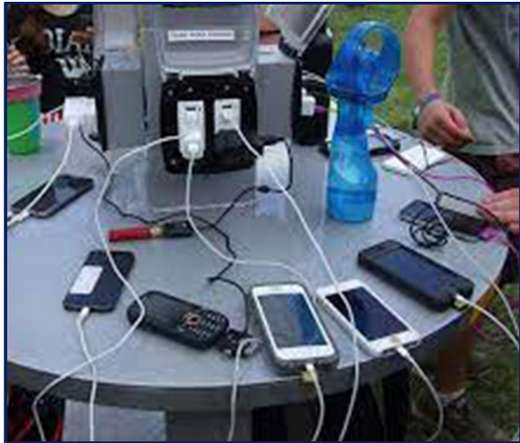
Charging stations / small battery distribution
